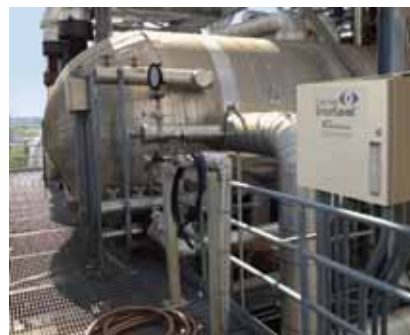
Control Unit shown with door-mounted SIS Series Indicator.
