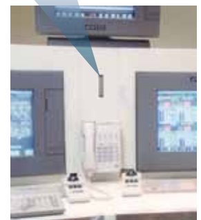
SIS Indicator in control room.
